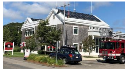
Oak Bluffs Fire Station
